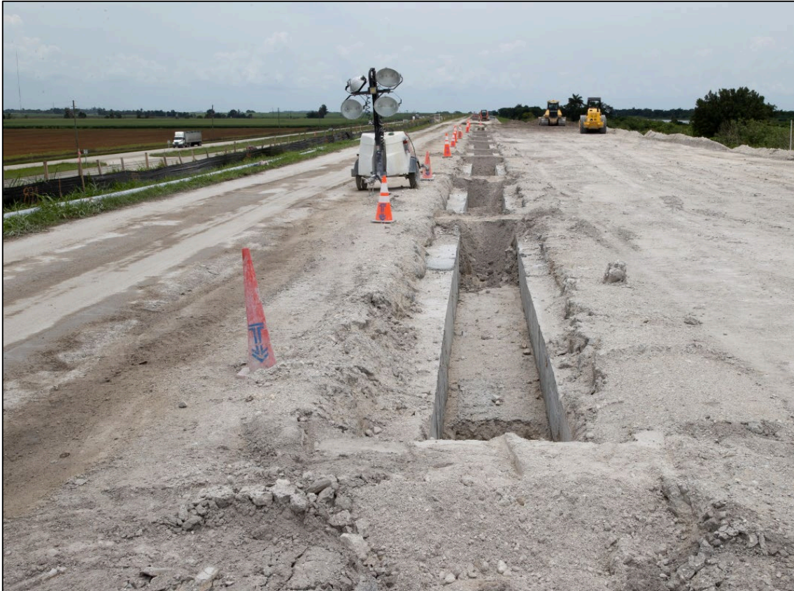
Cutoff Wall is Tested After 28-days and Accepted if Passes All Testing Criteria
