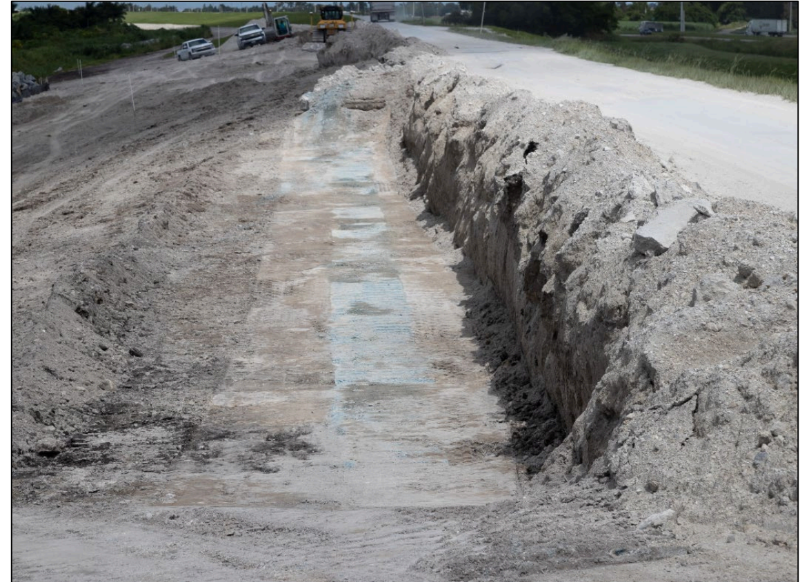
Concrete Guide Walls Removed and Embankment Restoration Begins
