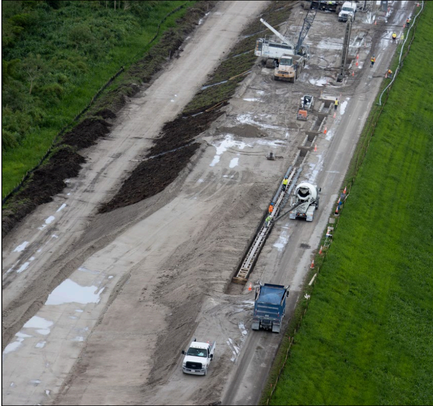
Concrete Guide Wall Construction
