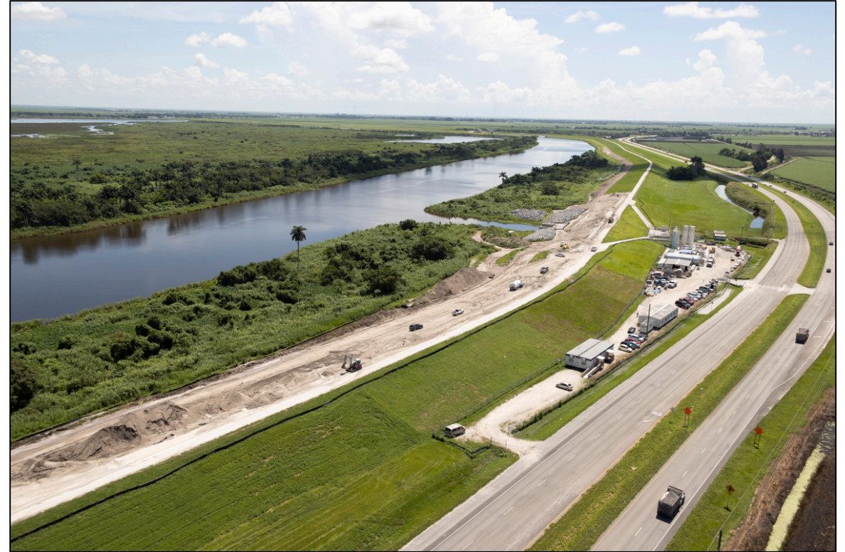
Work Platform Removal and Embankment Restoration
