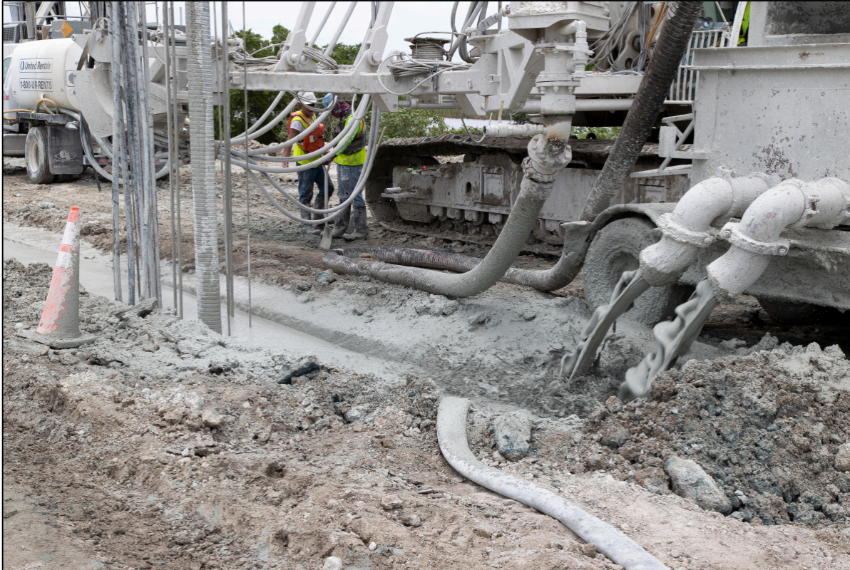
Hydromill Grinding through Rock to final Cutoff Wall Depth and Replaces Trench Slurry with Cutoff Wall Slurry
